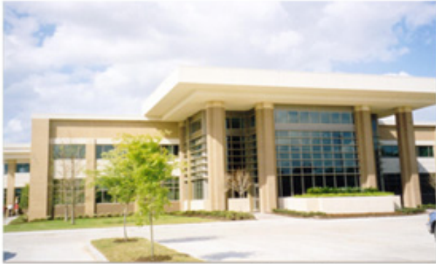
Louisiana Office of State Fire Marshal
